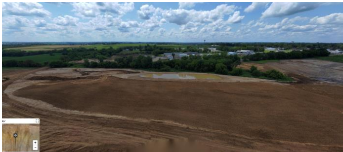
South Drainage Pond
