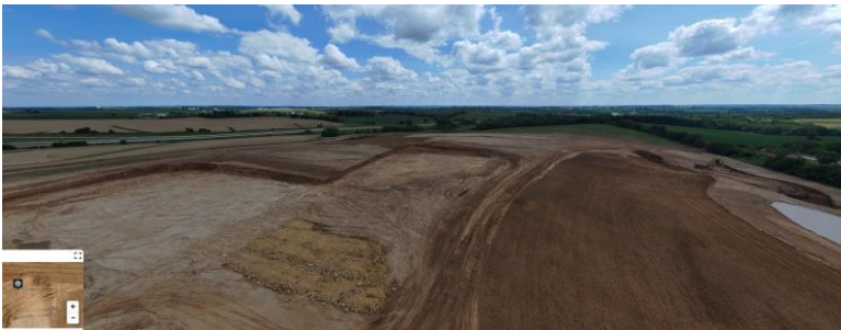
Building Footprint & West Parking Lot
